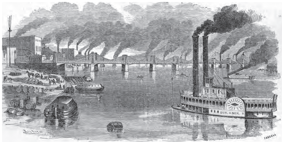
Mr. Kilbert and “Tarbell” (possibly Edmund N. Tarbell), A River Scene: Monongahela River, Pittsburgh, Pennsylvania . Shows steamship “General Knox,” wharf operations, a steel superstructure bridge, and numerous smoke stacks. Appeared in the Feb 21, 1857 edition of Ballou’s Pictorial . Reprinted from Wikimedia Commons.
